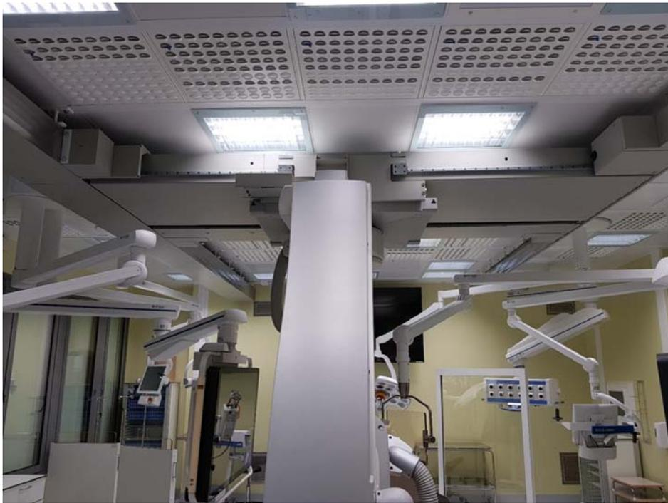
*Figure 1 Hybrid Operating Room in Nya Karolinska Hospital, Stockholm, Sweden, equipped with Halton Vita OR Space 5 ventilation system*
