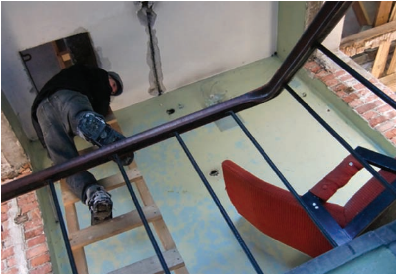
Figure 3. Ethnographic exploration of an abandoned house prior to its refurbishment. Narva Mnt. Tallinn, Estonia (Jan 2011, photo by Kerstin Kary)
