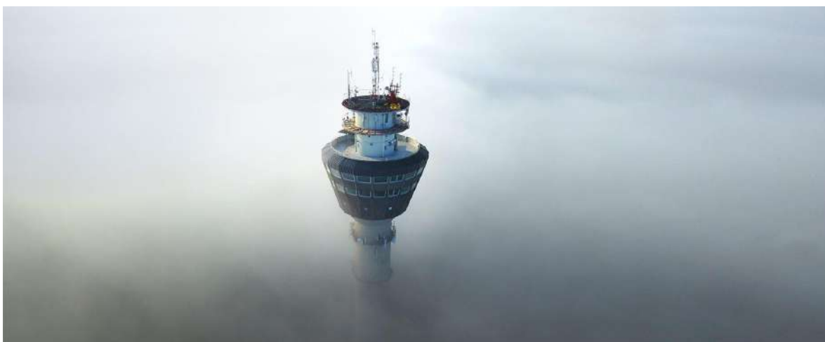
Figure 1. Puijo tower inside low-level clouds.
